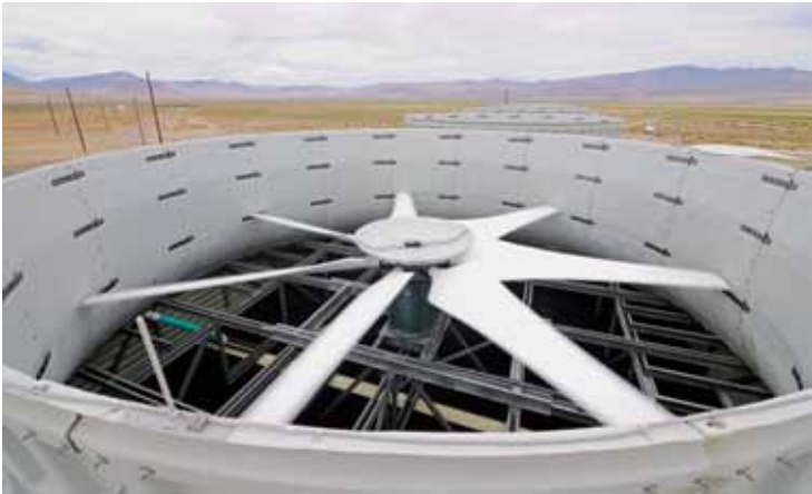
U.S. Geothermal also installed large-diameter fans and Baldor cooling tower motors at its San Emidio 9 net MW binary cycle power plant, located 100 miles northeast of Reno, Nevada.
