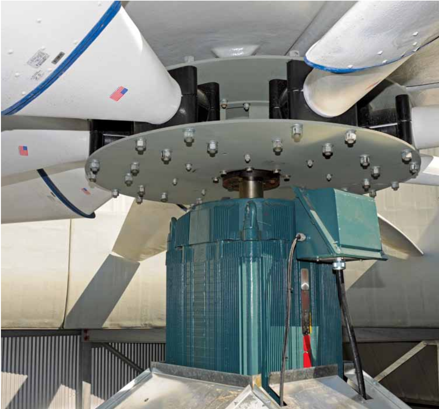
Baldor’s cooling tower motor is a high torque, direct drive motor specifically designed for cooling tower applications. The laminated finned frame construction provides a highly efficient, power-dense package that replaces the right angle gearbox and jack shaft installation found in conventional cooling towers. The fan couples directly to the motor shaft and is controlled by Baldor’s VS1 cooling tower drive.
