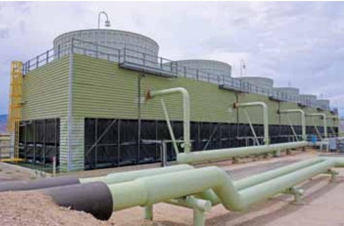
U.S. Geothermal also installed large-diameter fans and Baldor cooling tower motors at its San Emidio 9 net MW binary cycle power plant, located 100 miles northeast of Reno, Nevada.
